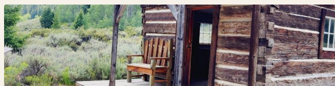
CHINKED LOG AND A PLANK PORCH ON THE TOWNSITE
